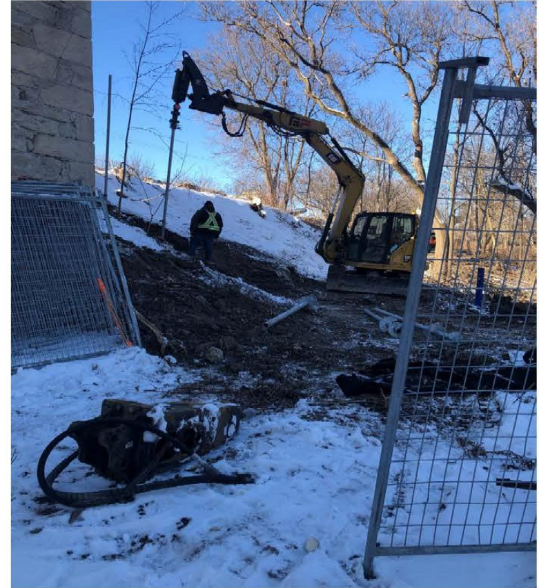
Photo #2: Helical pile installation completed.
