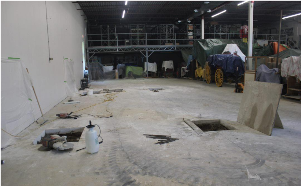
Cutting new footings (above) and newly poured footings (below) for mezzanine expansion.
