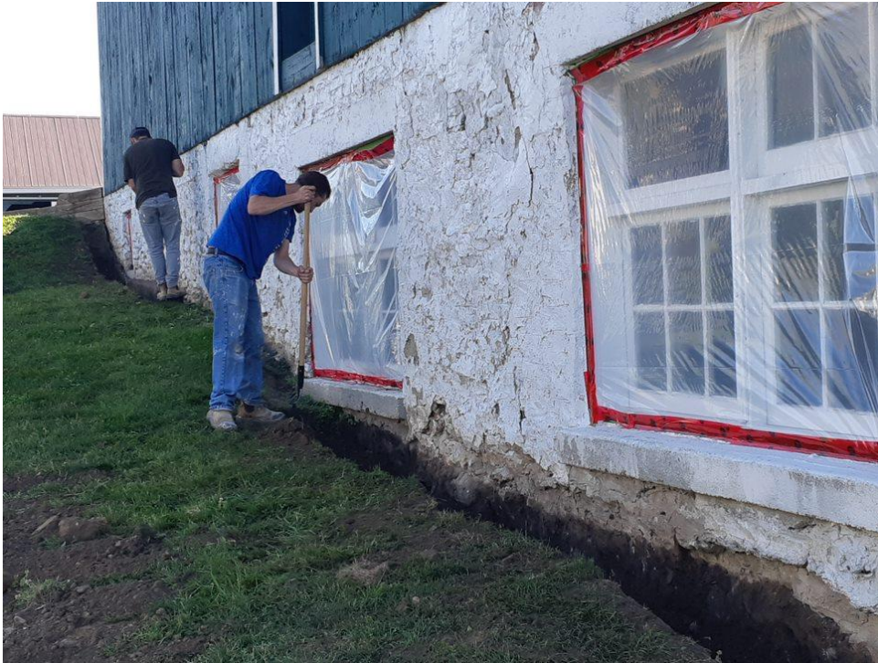
West wall of stable prior to removal of paint and old mortar (August 2022).
